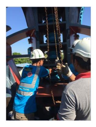
Replacement of TBM cutter disc
